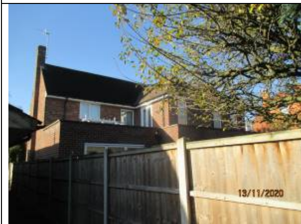
Rear elevation of 34 Park Road
