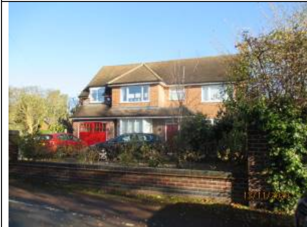
Front elevation of 34 Park Road
