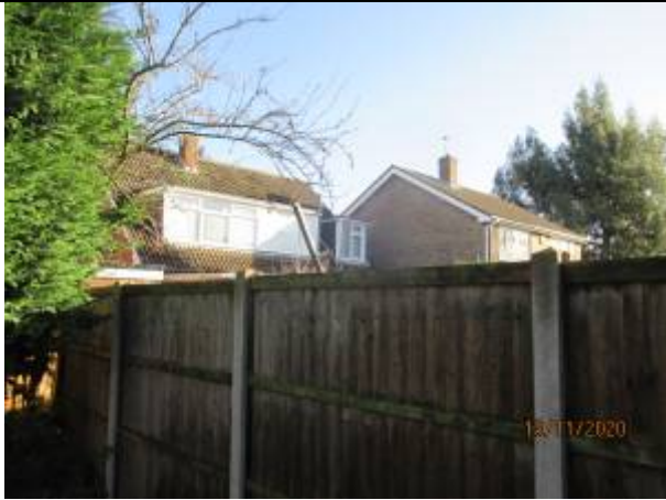
Rear elevation of 2 Rookwood Close
